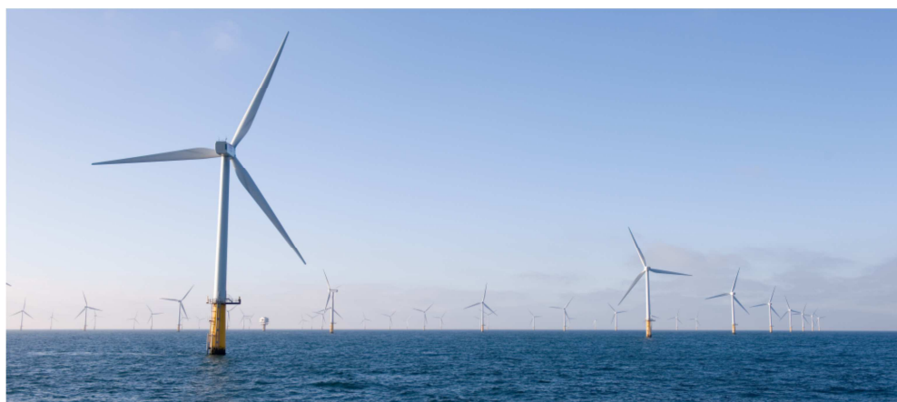
Figure 1.1 Overview of Princess Amalia Offshore Wind Farm [ref. beeldbank.rws.nl].
