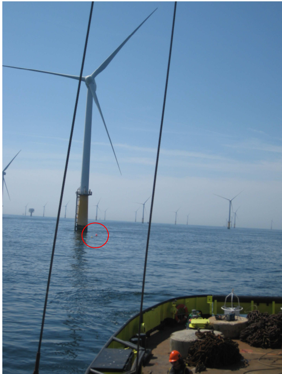
Figure 3.4 Deployment and recovery vessel 'Terschelling' near WTG1 Vestas V80 turbine. The orange and yellow floats, within the red circle, indicate position H1 with Sesame deployed.
